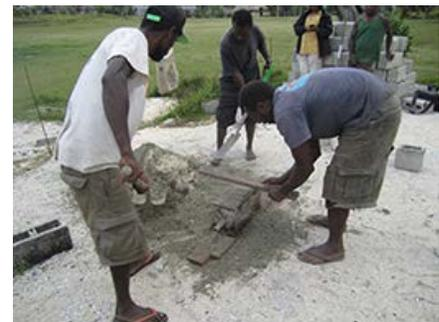
The community are continuing the production of concrete blocks, to be used in the construction of the bungalow wet areas and water tanks.
