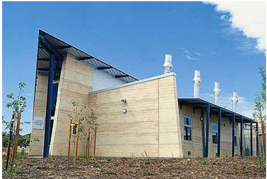
Sound construction: Playford Primary School's environmentally friendly building
