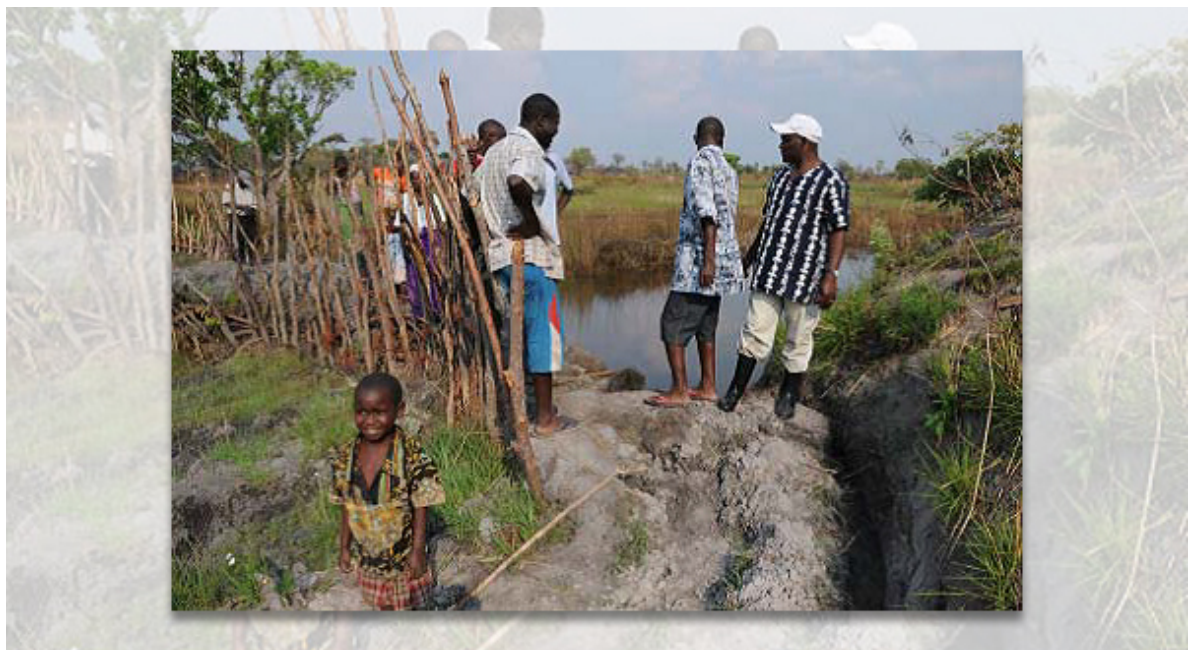
Image: Irrigation furrow is clogged during night time, so that water is stored in the pond formed with the weir. With the stored water, farmers could extend irrigation to more farmlands.
