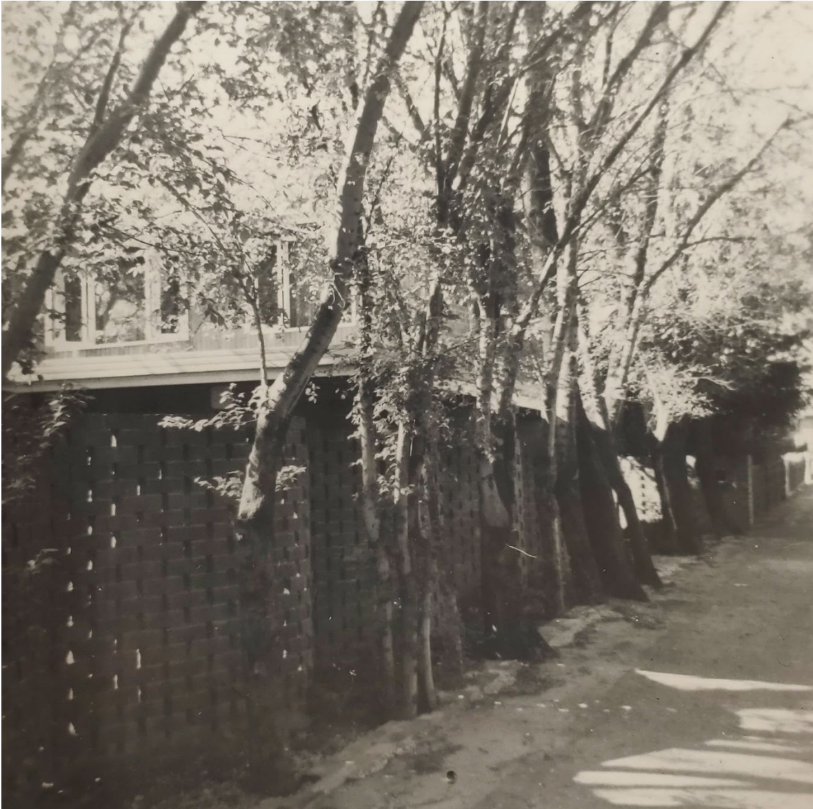
110 George Street, Norwood, Brian Polomka, 1954-64, Polomka collection, Architecture Museum, University of South Australia.
