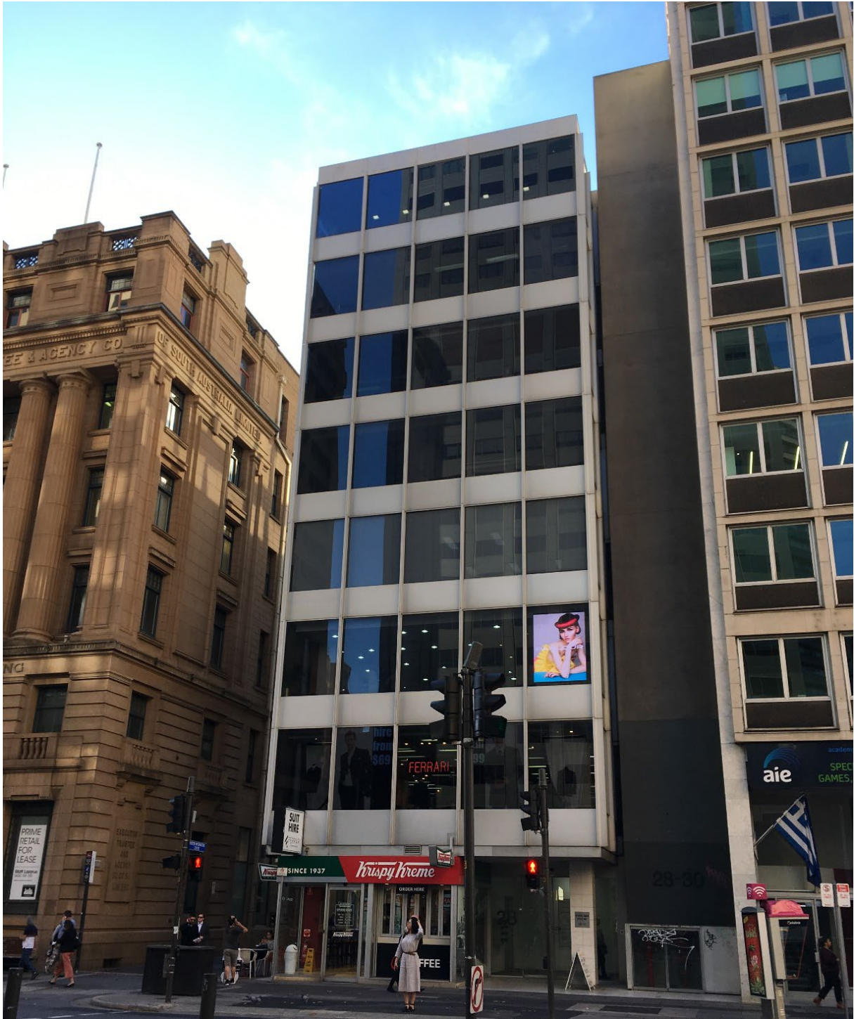
Eagle Star Insurance Building, Grenfell Street, Adelaide, photograph Louise Bird.
